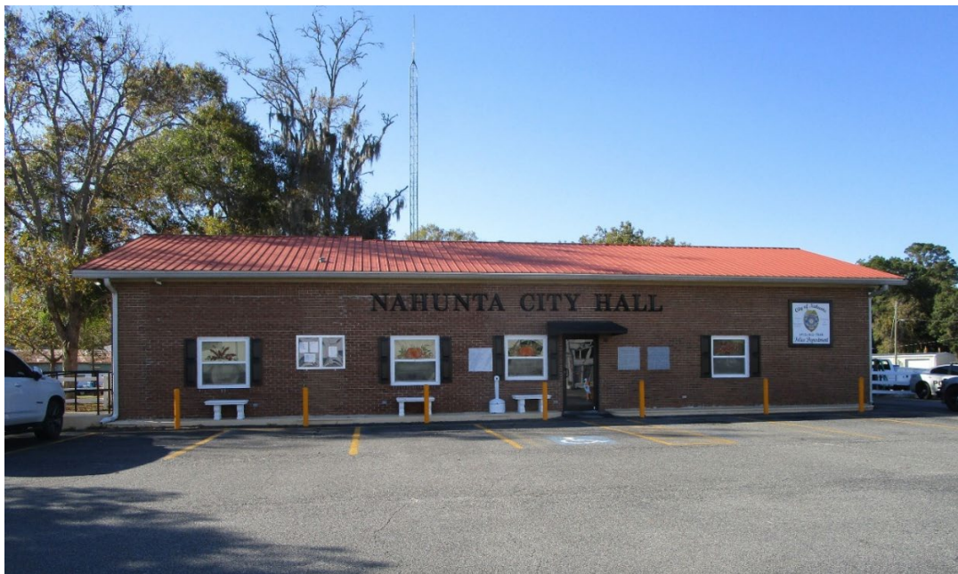
Nahunta City Hall and Police Department
